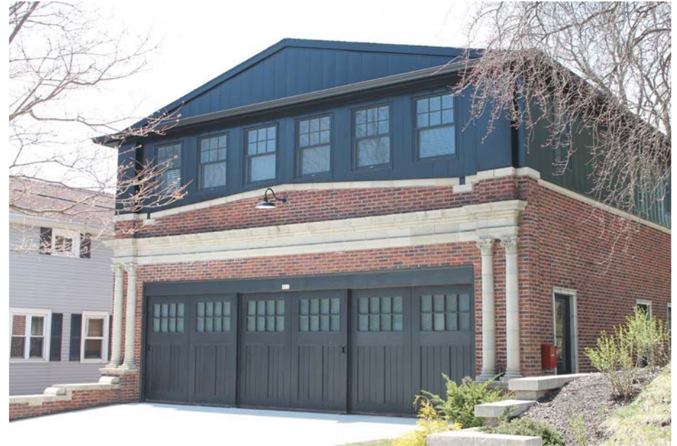
NOT RECOMMENDED new construction negatively impacting a building's character
