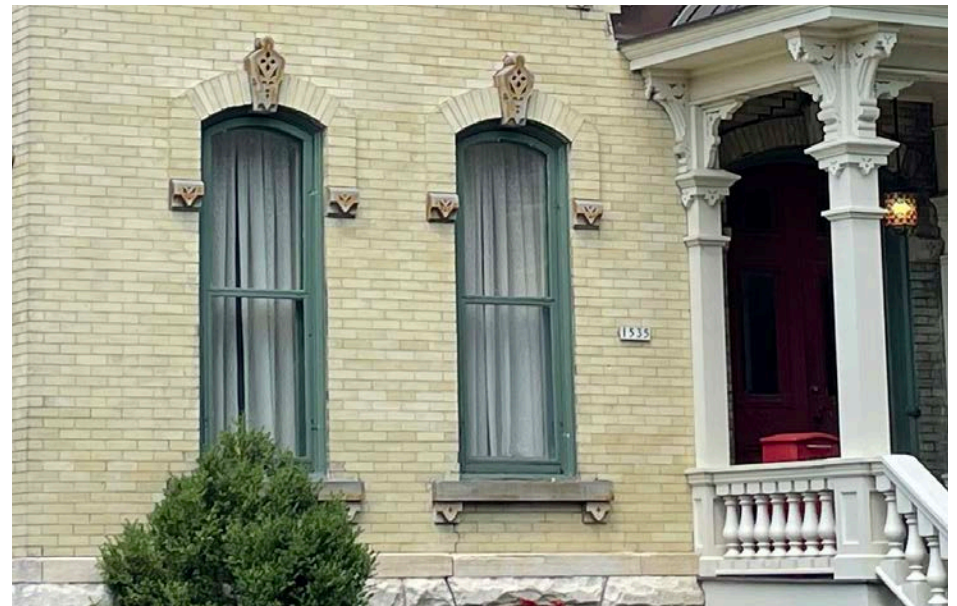
RECOMMENDED for wood double hung windows, stone sills, and brick window hoods.
