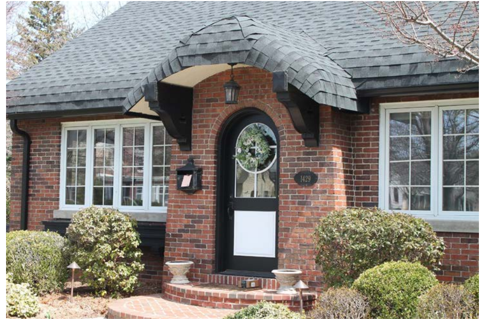
RECOMMENDED retaining and maintaining original light fixtures
