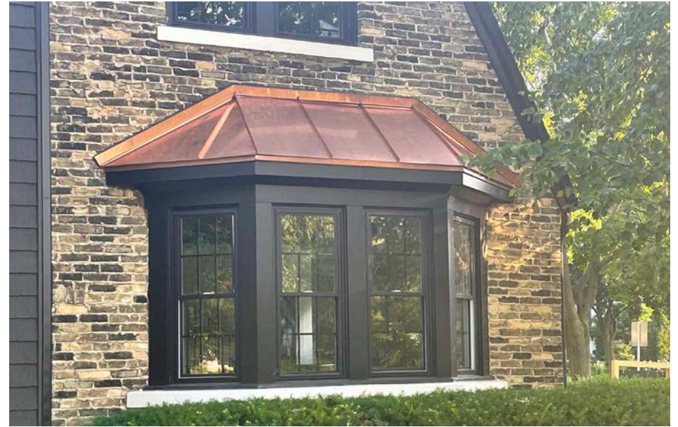
RECOMMENDED Replacing a metal feature in kind or with a compatible substitute
