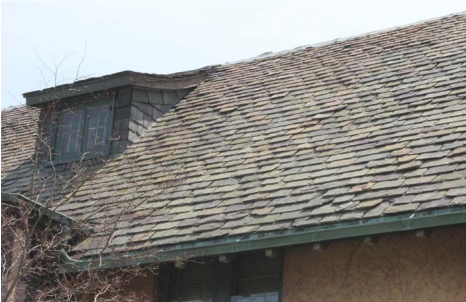
RECOMMENDED retaining and maintaining slate roof and dormer
