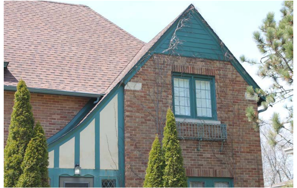
RECOMMENDED retaining wood siding and decorative features
