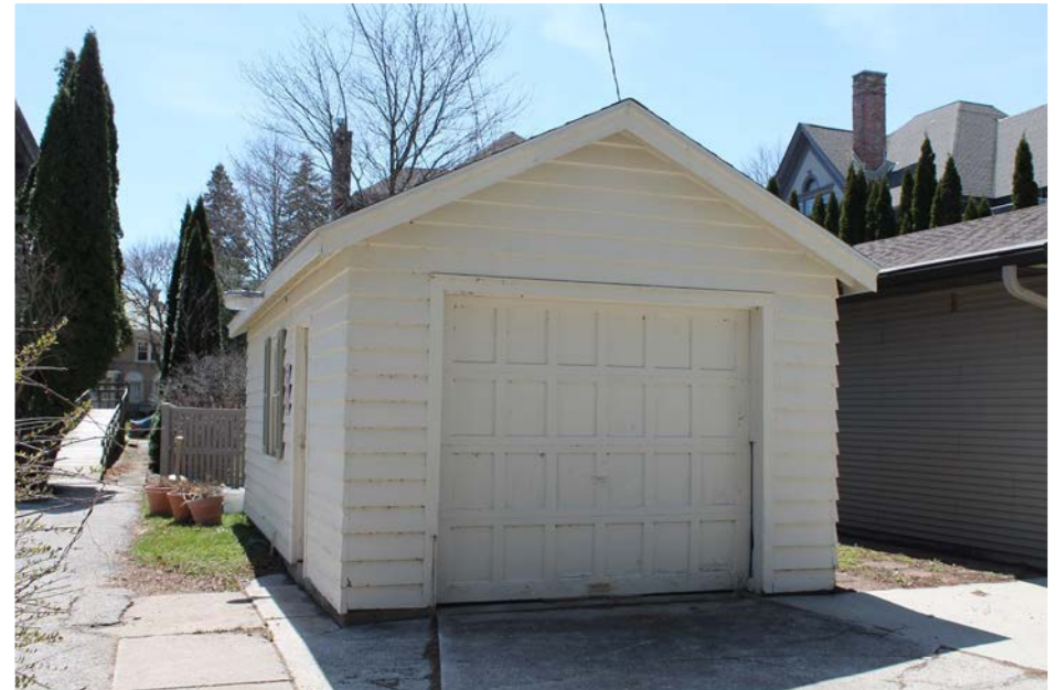
RECOMMENDED retaining and maintaining original accessory structures
