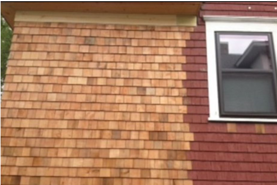
RECOMMENDED replacing wood shingles in kind (photo taken prior to painting)
