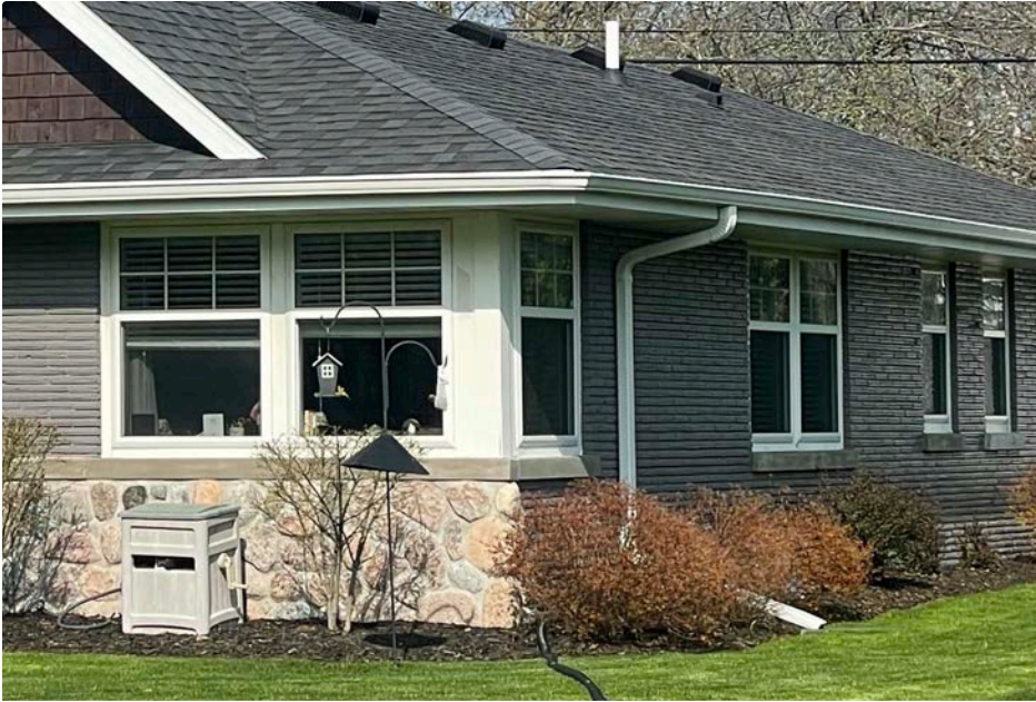
NOT RECOMMENDED vinyl windows with window grids in incompatible style for house
