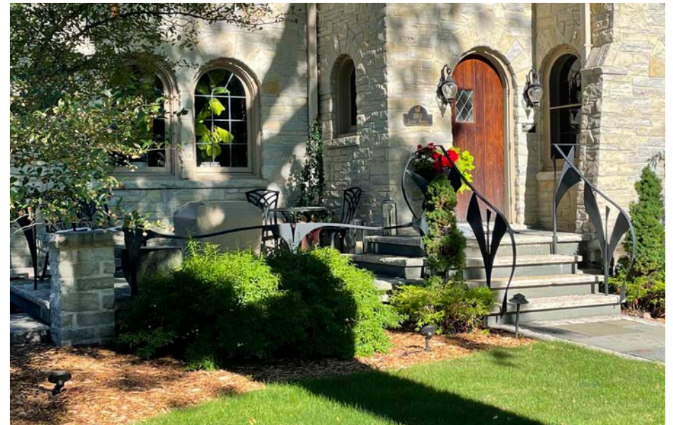
NOT RECOMMENDED decorative wrought iron railings visible from the street
