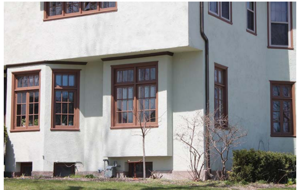
RECOMMENDED repairing and patching stucco with new to duplicate the old
