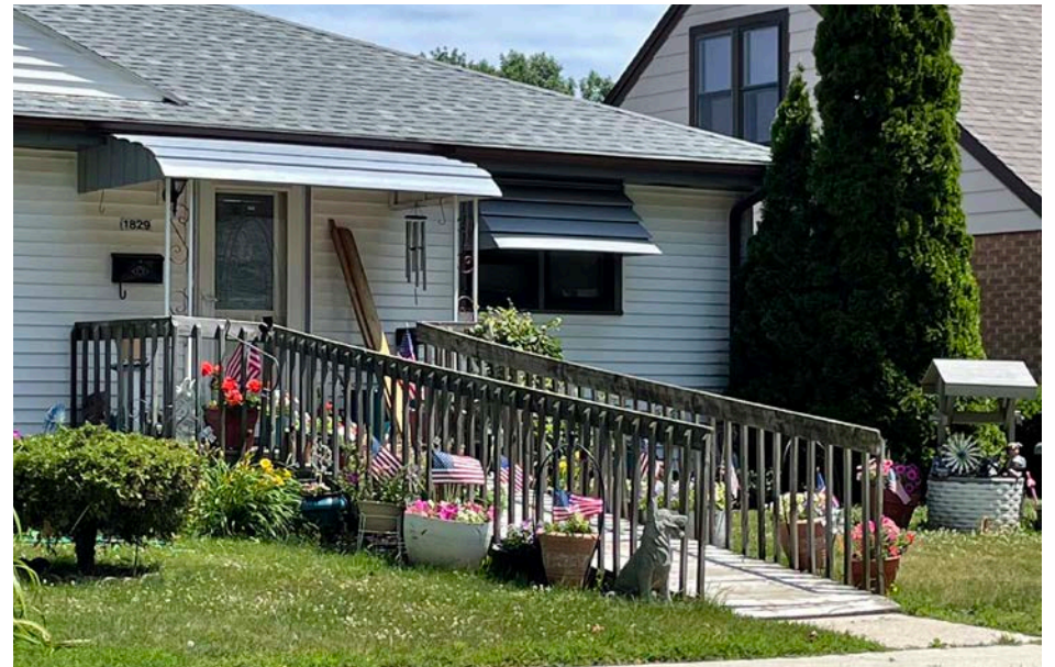
NOT RECOMMENDED installing incompatible ramps at a primary entrance
