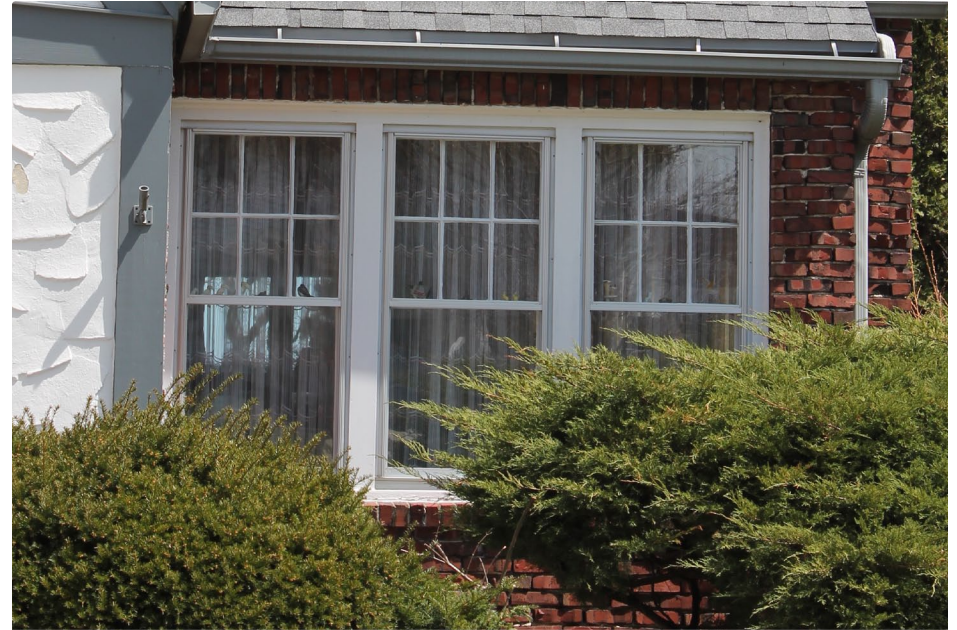
RECOMMENDED retaining and maintaining multi-lite wood double hung windows.
