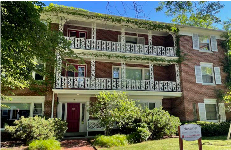
RECOMMENDED applying appropriate paint to historically coated metal features
