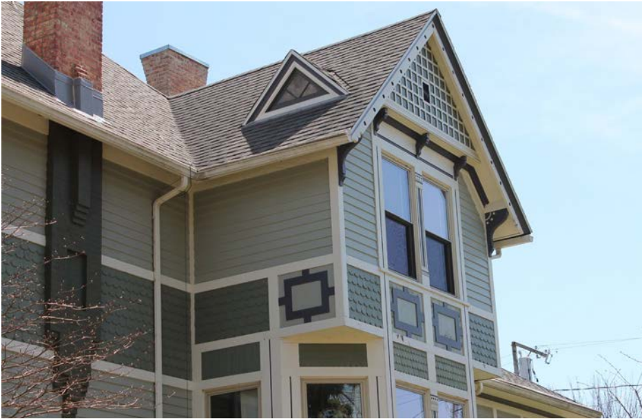
RECOMMENDED retaining and maintaining wood siding and decorative features
