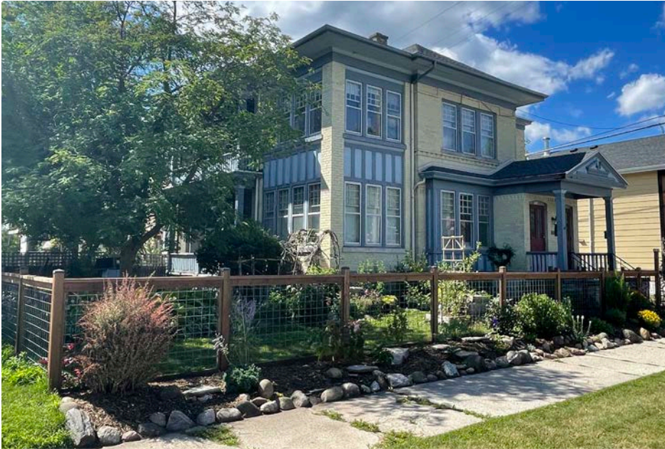
NOT RECOMMENDED incompatible fencing that negatively impacts historic character
