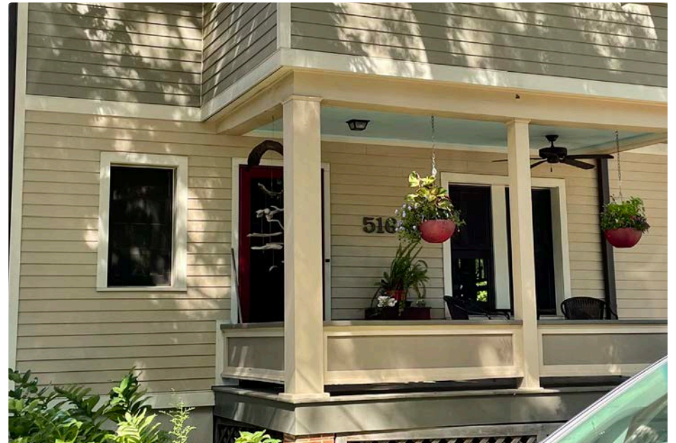
RECOMMENDED replacing with a compatible new substitute material similar to the old
