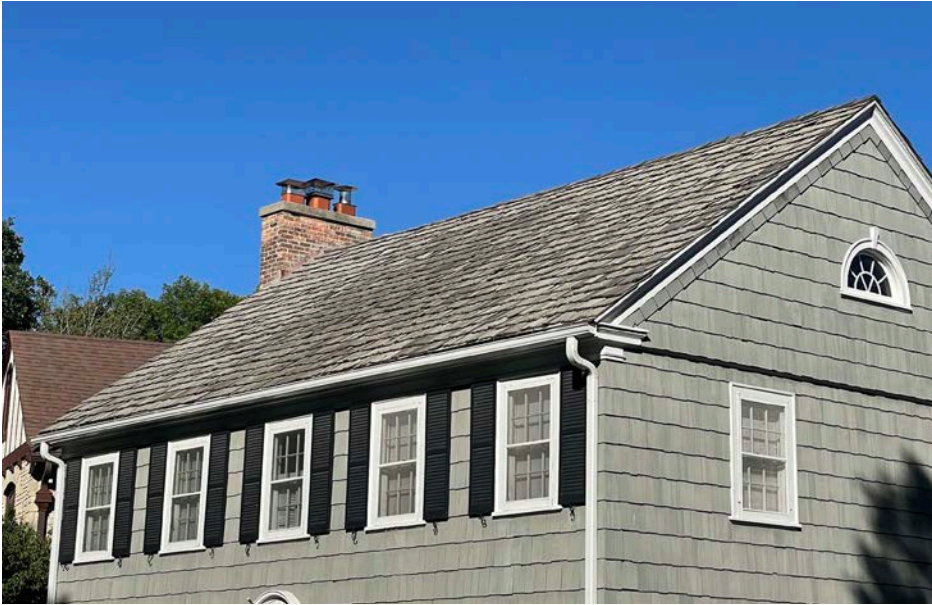
RECOMMENDED retaining wood shingle roof, returned eaves, and masonry chimney
