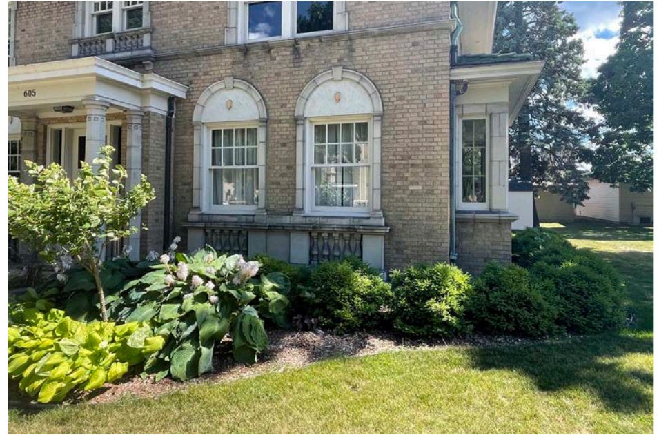
RECOMMENDED maintaining drainage to ensure water does not damage features
