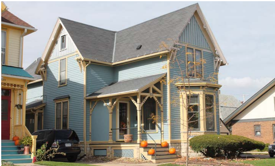
(ABOVE) 914 Lake Avenue , (OPPOSITE PAGE) 400 7th Street
