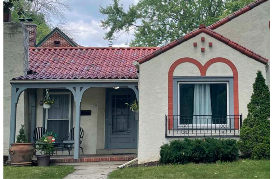
NOT RECOMMENDED replacing two double hung windows with single fixed window
