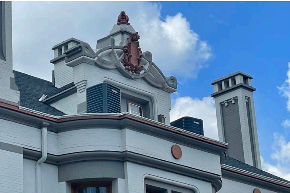
NOT RECOMMENDED placing rooftop equipment visible from the street
