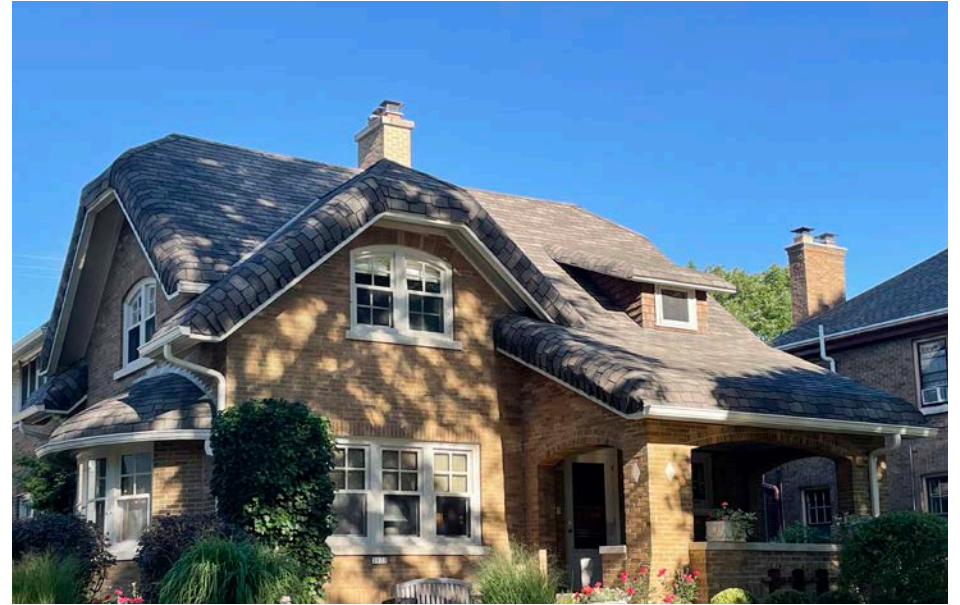
RECOMMENDED retaining roof form with new replacement asphalt shingle roofing
