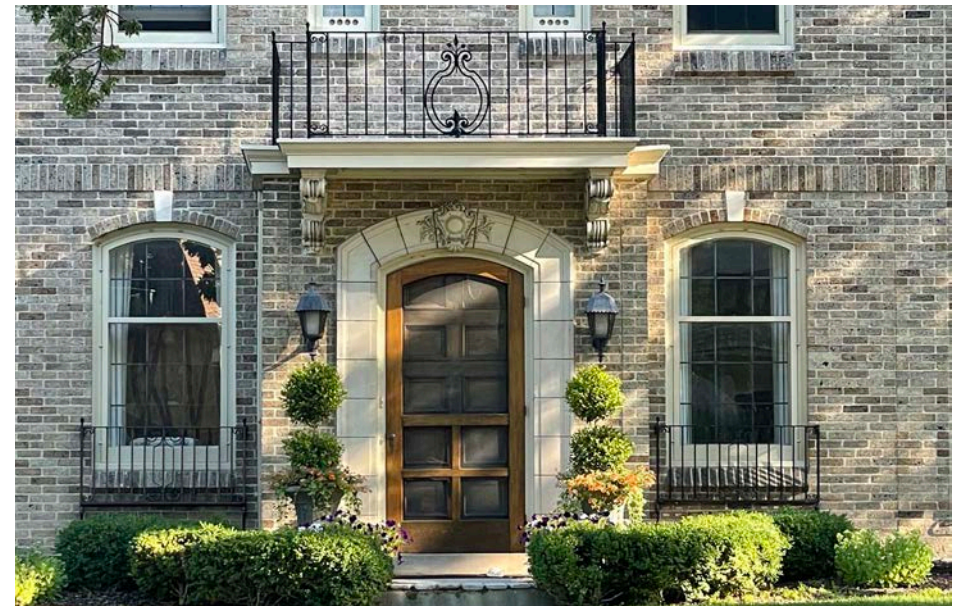
RECOMMENDED retaining and maintaining decorative wrought iron features
