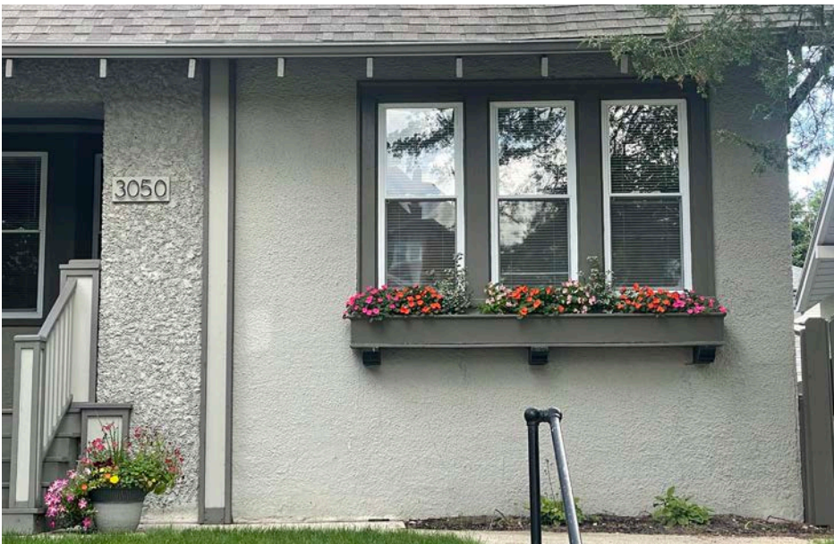
NOT RECOMMENDED patching stucco with new that does not duplicate the old
