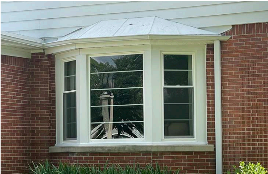
NOT RECOMMENDED applying paint to a metal feature that was not coated historically
