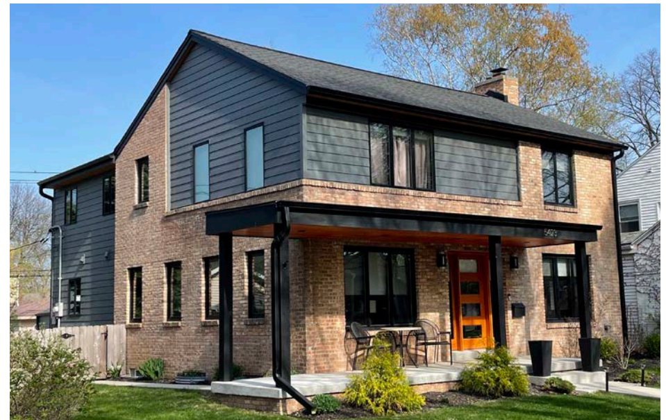
NOT RECOMMENDED additions and alterations significantly different from historic house
