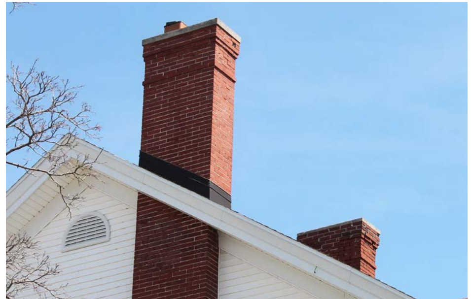
RECOMMENDED retaining and maintaining chimney cap and decorative features
