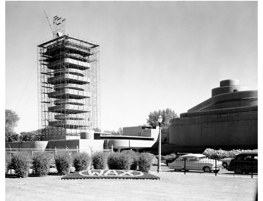
The Frank Lloyd Wright designed Johnson Wax Research Tower under construction.
