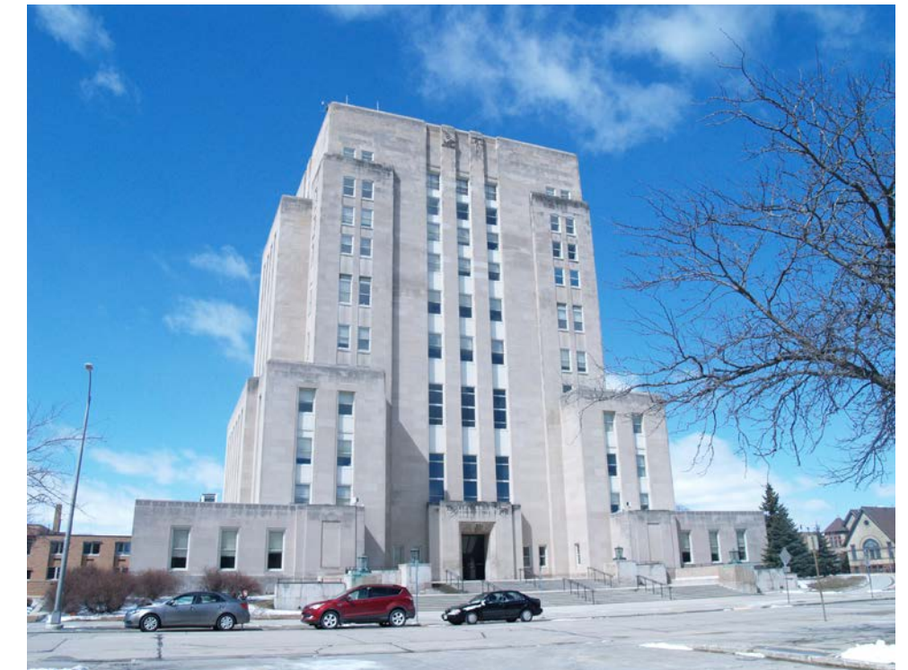
Racine County Courthouse - 730 Wisconsin Avenue
