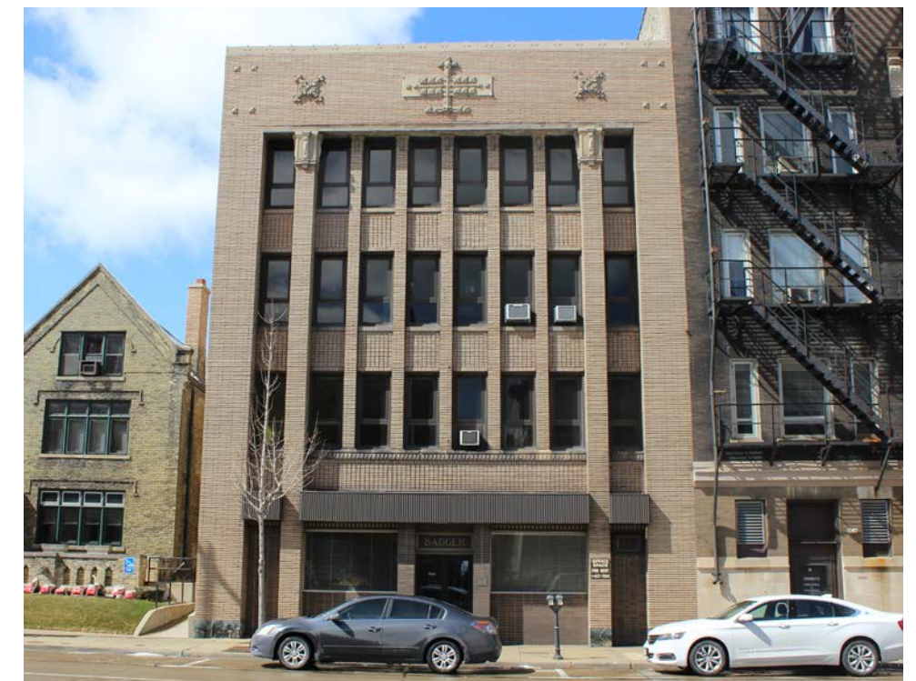
Badger Building - 610 Main Street
