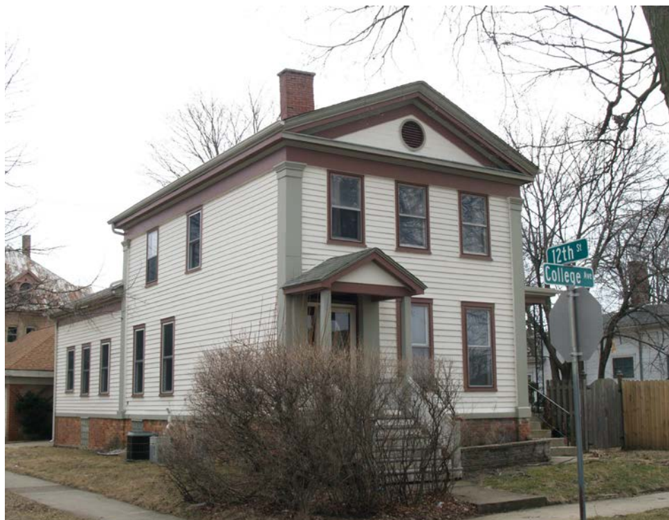
Greek Revival - I-Shaped Cottage at 12th and College.
